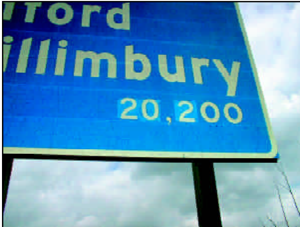
Figure 4.10A Overlay Sheet on Extruded Panel Sign
