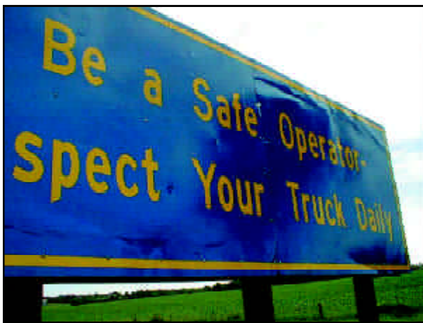
Figure 4.10B Overlay Sheet on Extruded Panel Sign
