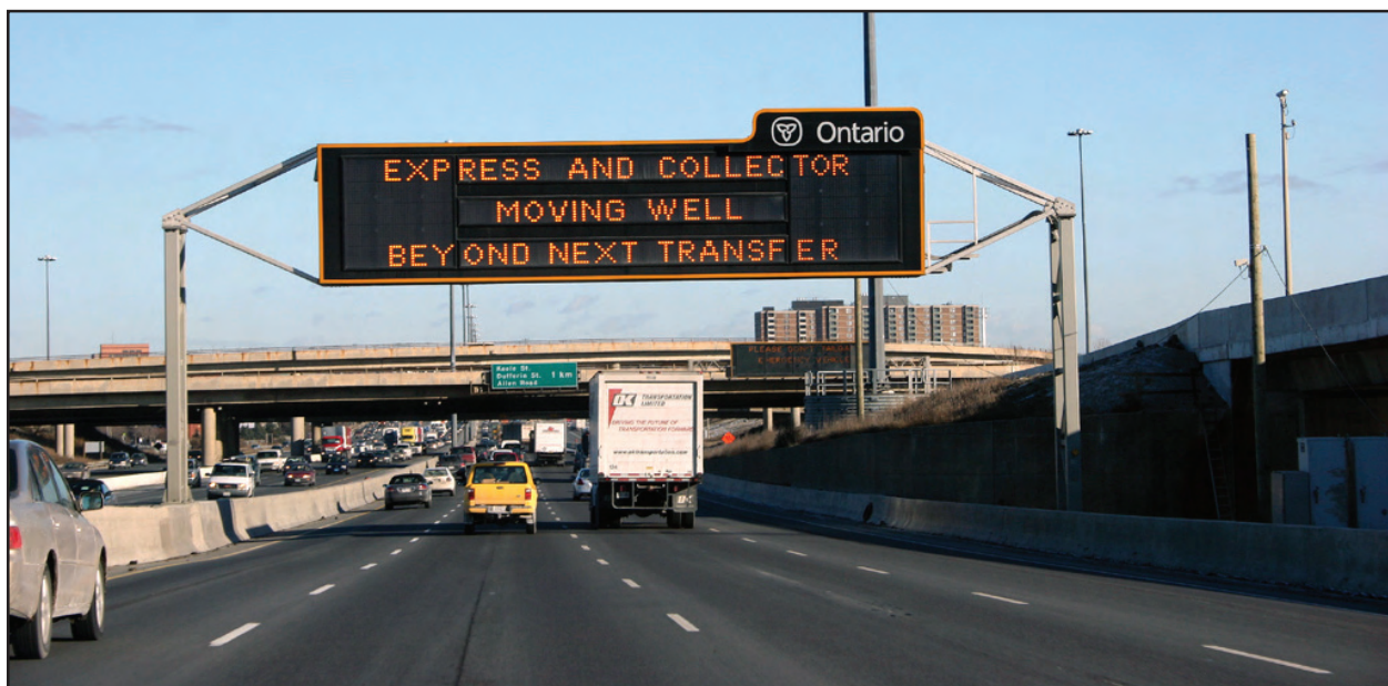
Figure 12 – MTO Overhead Gantry-Mounted DMS
