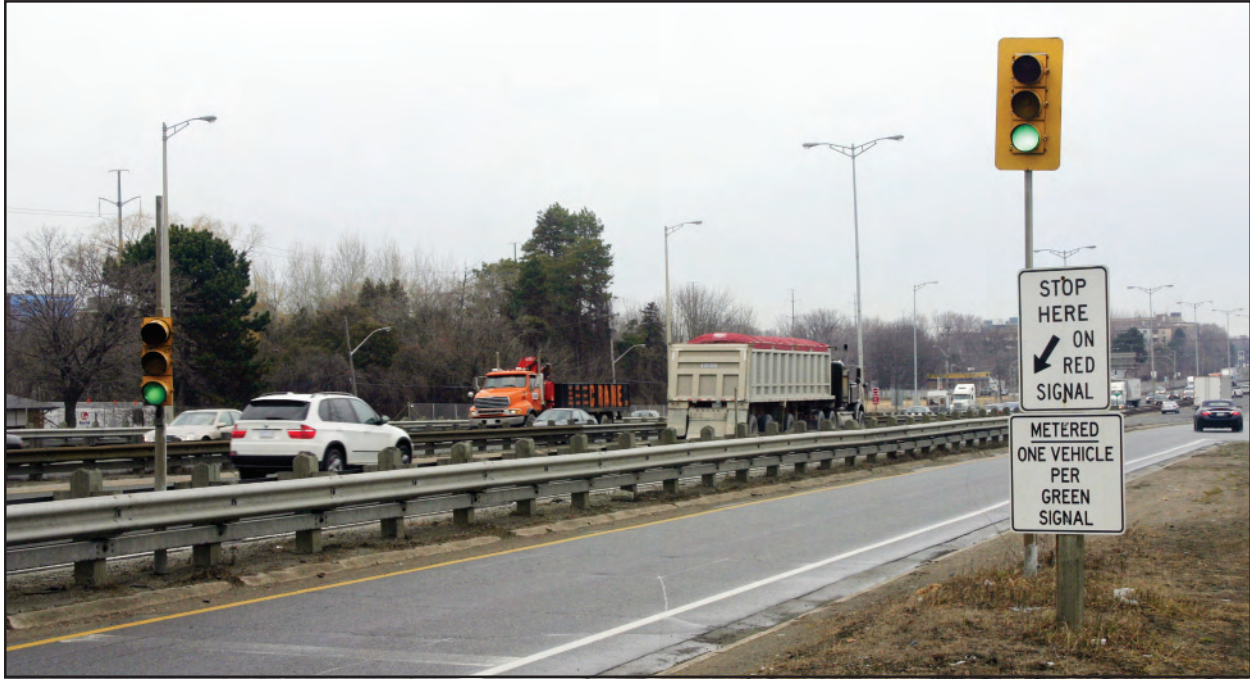
Figure 11 – Signals for Ramp Metering
