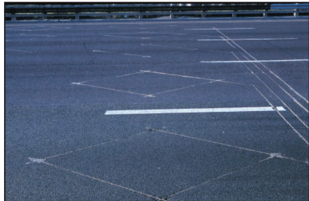
Figure 3 – Typical Inductive Loop Arrangement
